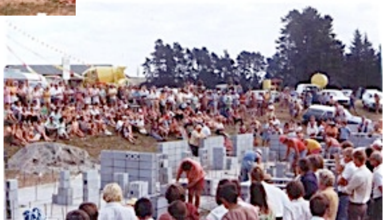
A Blocklaying Competition at the 1975 NZ Building & Construction Fieldays produced a toilet block for future use at Mystery Creek. (See appropriate chapters for details on NZ Building Fieldays activities).
